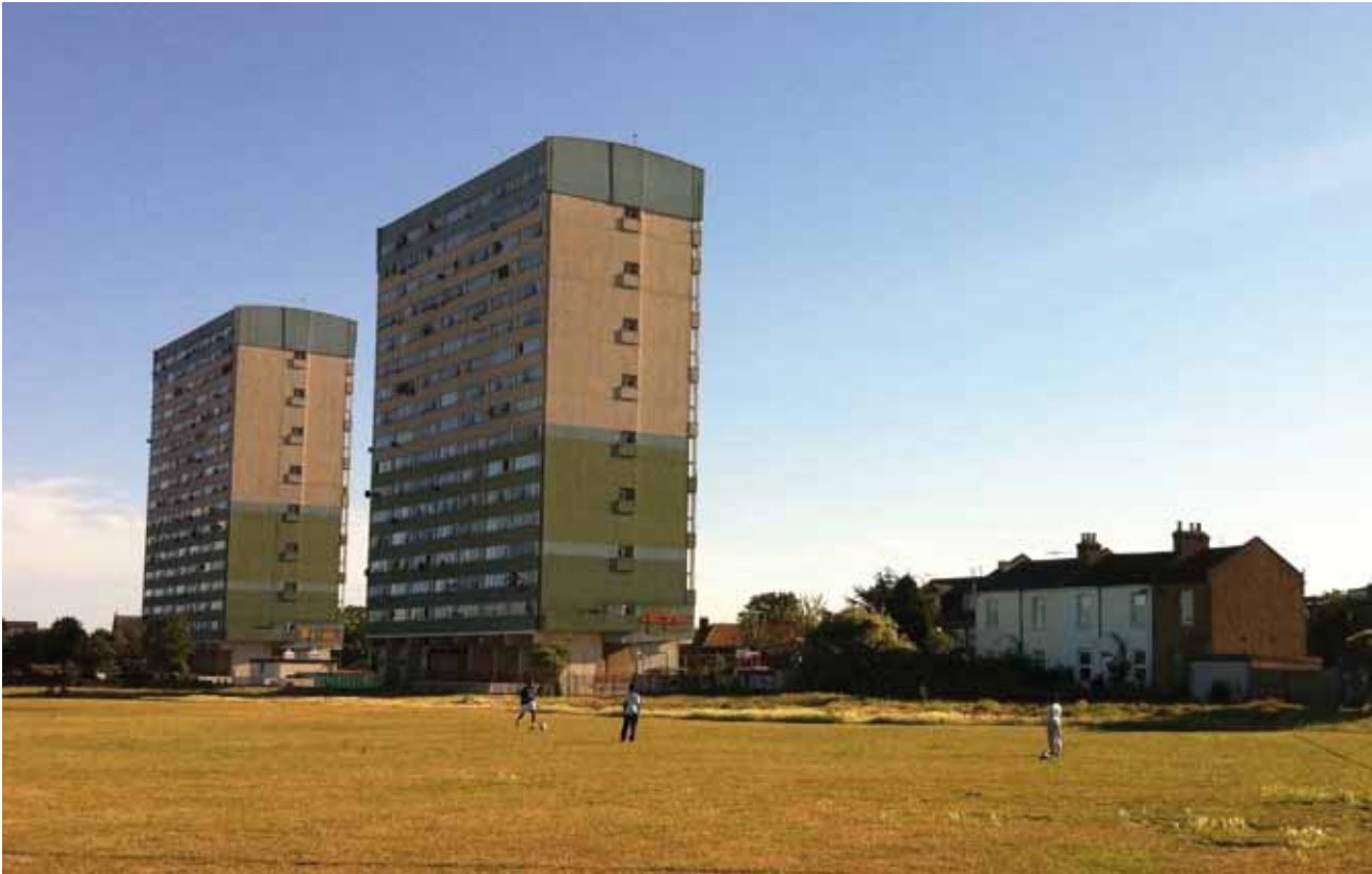
Figure 5: Poorly built 1960s blocks over looking Wanstead Flats, London. Fungus, cracked walls and overflowing sewage prompted irate tenants from neighbouring blocks to invade their local town hall to complain; at the time, their homes were just four years old
