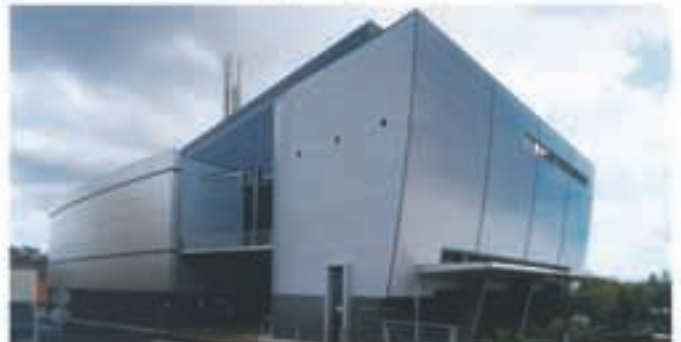
Princess Alexandra Hospital, Brisbane, Australia
