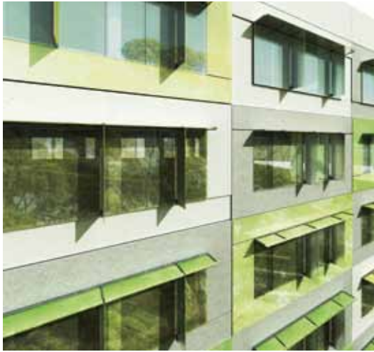
Detail of inpatient unit cladding showing coloured and patterned, glazed sunshading system
