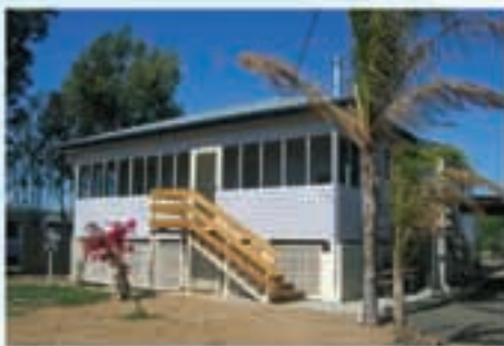
Goodooga Community Housing Project, New South Wales, Australia
