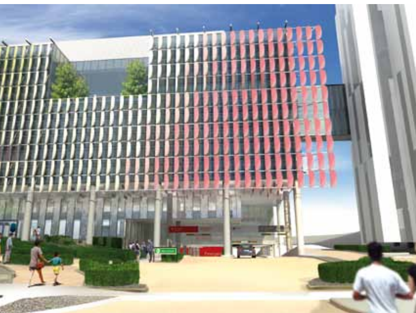
View of the front facade showing array of coloured glass blades
