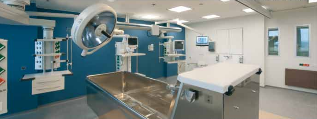
MILITARY HOSPITAL in Brussels, Belgium | European Reference Center for Burns treatment | delivery autumn '09
