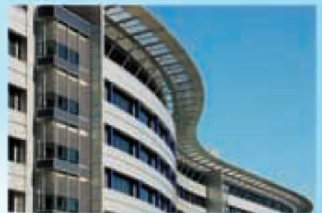
Princess Alexandra Hospital, Brisbane, Australia
