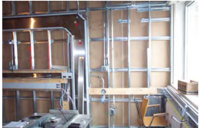
Wall-mounted biomedical raceway
