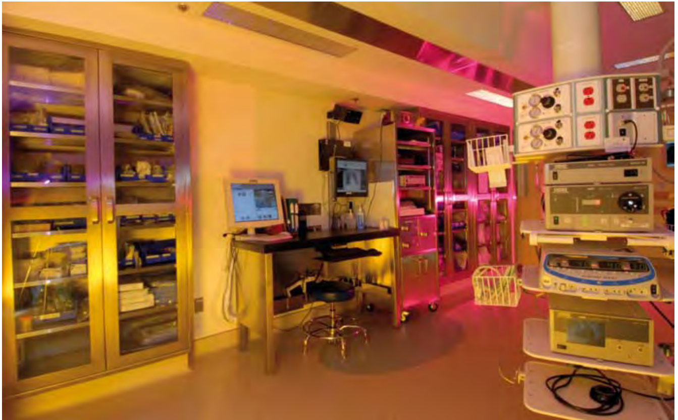
Ceiling biomedical raceway
