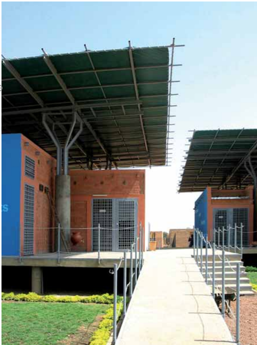
The centre is set atop a raised platform to ensure hygienic/climatic conditions
