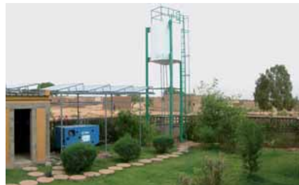
Photovoltaic cells have been installed along the perimeter wall
