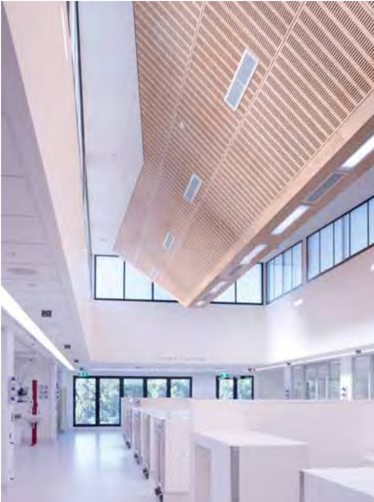
Large roof lanterns and switchable glass fill the Alfred ICU in Melbourne with natural daylight
