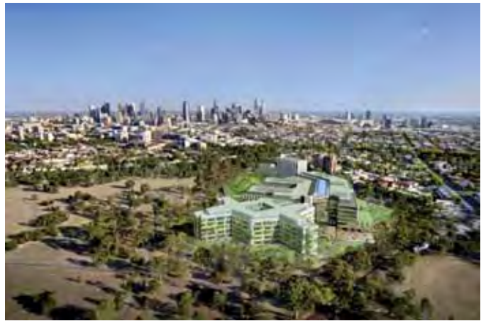
Royal Children's Hospital in Melbourne takes advantage of local parkland in its design
