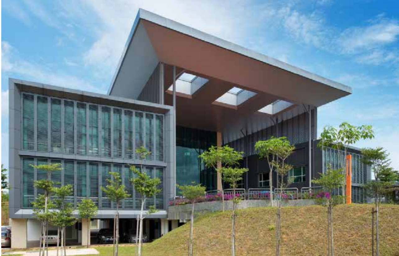
Socso Rehabilitation Centre Administration Block
