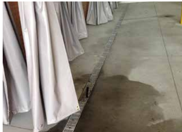
Fig. 3 b: Decontamination Shower Trench Drain
