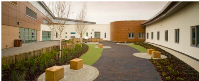
Safevent windows were installed at Discovery House in Lincoln
