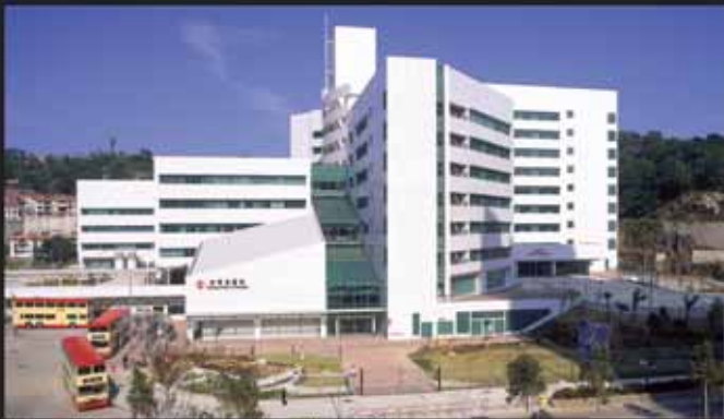
Tseung Kwan O Hospital, Hong Kong, China
