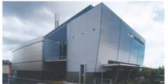
Princess Alexandra Hospital, Brisbane, Australia
