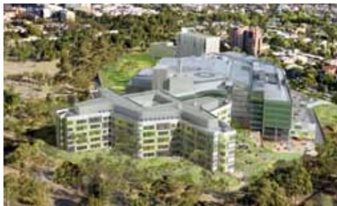
The hospital in the city: the new Royal Children's Hospital, Melbourne
