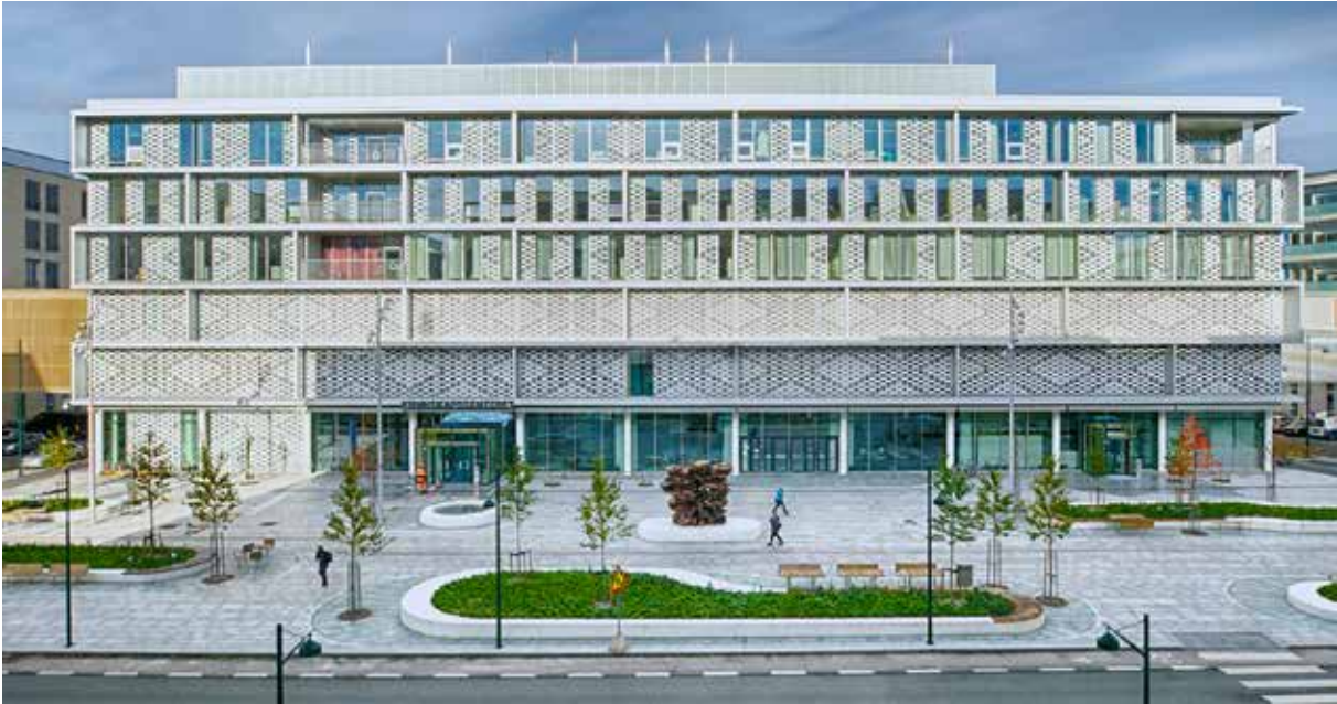
Wellness center at the Trondheim Hospital, Norway
